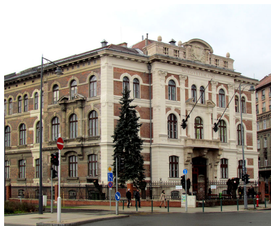
Fig. 10 The chemistry building “CH” of the Budapest University of Technology and Economics, 4 St. Gellért Square, District XI (it was built in 1902 and houses about half of the chemistry faculty). Photograph by the author
